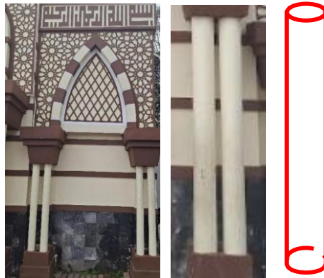
Figure 9. Cylindrical Supporting Pillar
