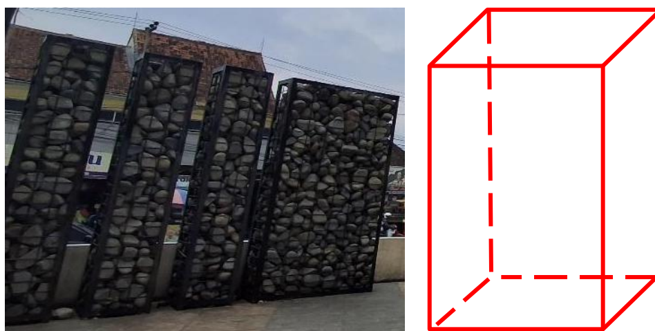
Figure 10. Gabion Fence in the Form of a Rectangular Prism
