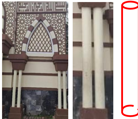
Figure 9. Cylindrical Supporting Pillar
