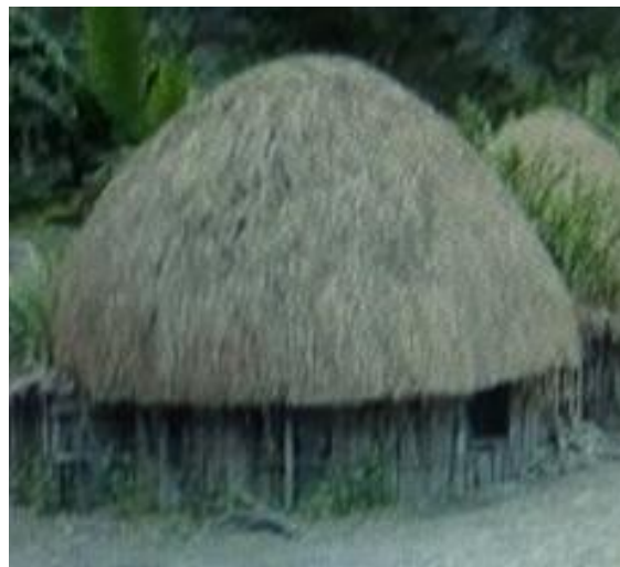
Figure 13. The paraboloid roof
