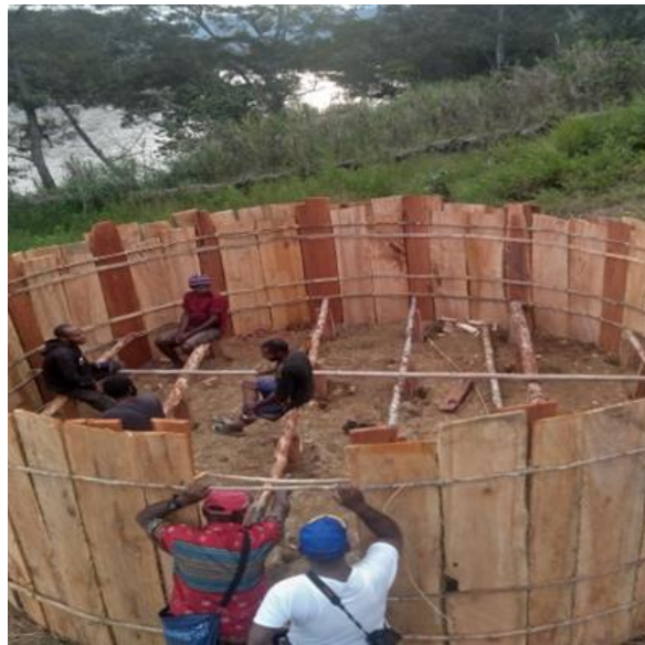
Figure 6. Construction of the lower floor of the Honai
