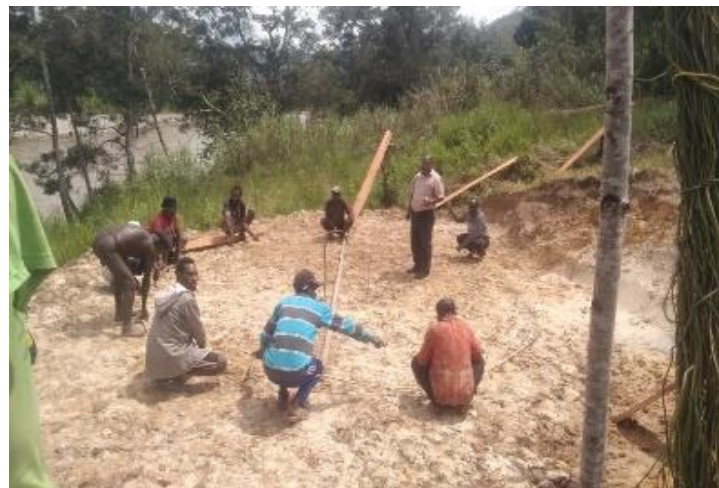
Figure 3. Making a bare circle of Honai using rattan
