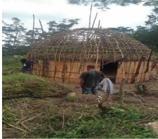
Figure 9. Installation of the roof frame
