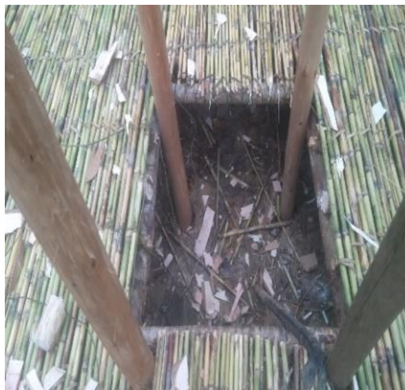
Figure 7. Installation of the four main pillars
