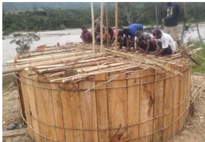
Figure 8. Construction of the upper floor of the Honai
