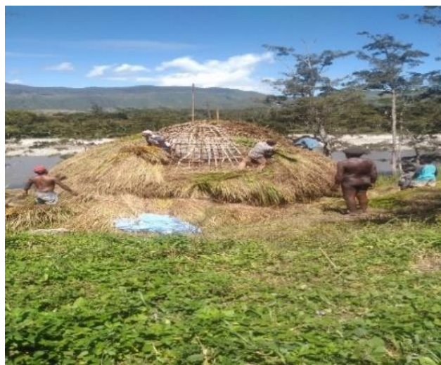
Figure 10. Covering the roof with thatch
