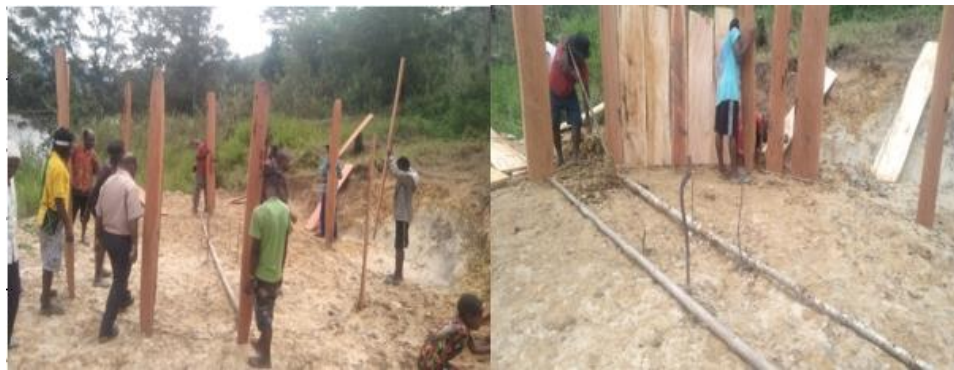
Figure 4. Installation of wooden planks around the circular base of the Honai
