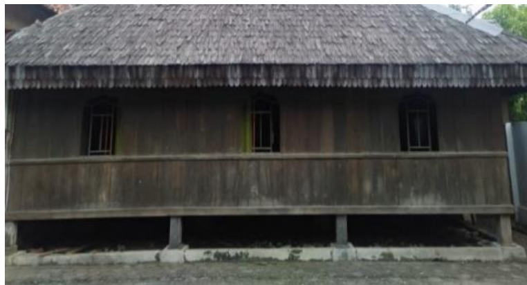
Figure 3. Darussajidin Mosque Wall and Air Vents
