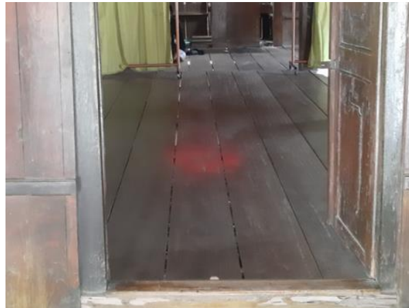
Figure 6. Darussajidin Mosque Floor
