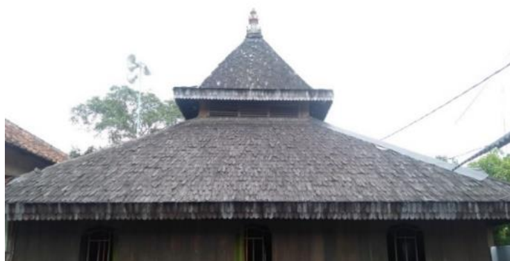
Figure 1. The Roof of the Darussajidin Mosque
