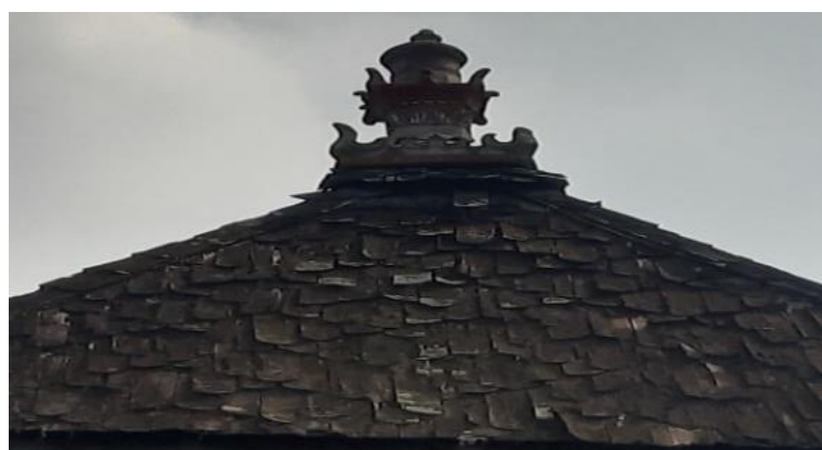
Figure 2. Dome of Darussajidin Mosque
